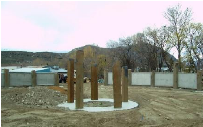
All eight of the plaque walls are now in place.
